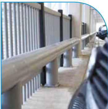
Car Park Barrier with Anti-Climb
